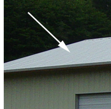
Non-Painted Roof (Galvanized)
